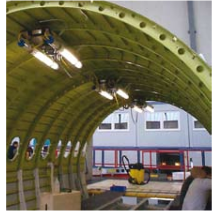
Safety tubular lights 975 used in airplane maintenance in the Airbus.
